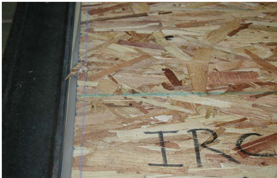
Figure 3. IRC panel specimen (nominal 8 ft opening span) showing pull-thru and edge tear-out of one #8 screw at one end of the panel.
